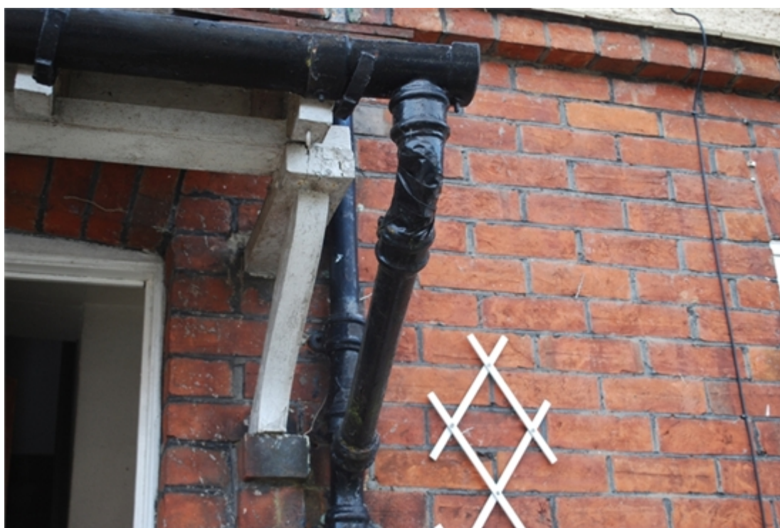
Downpipe taped together.
