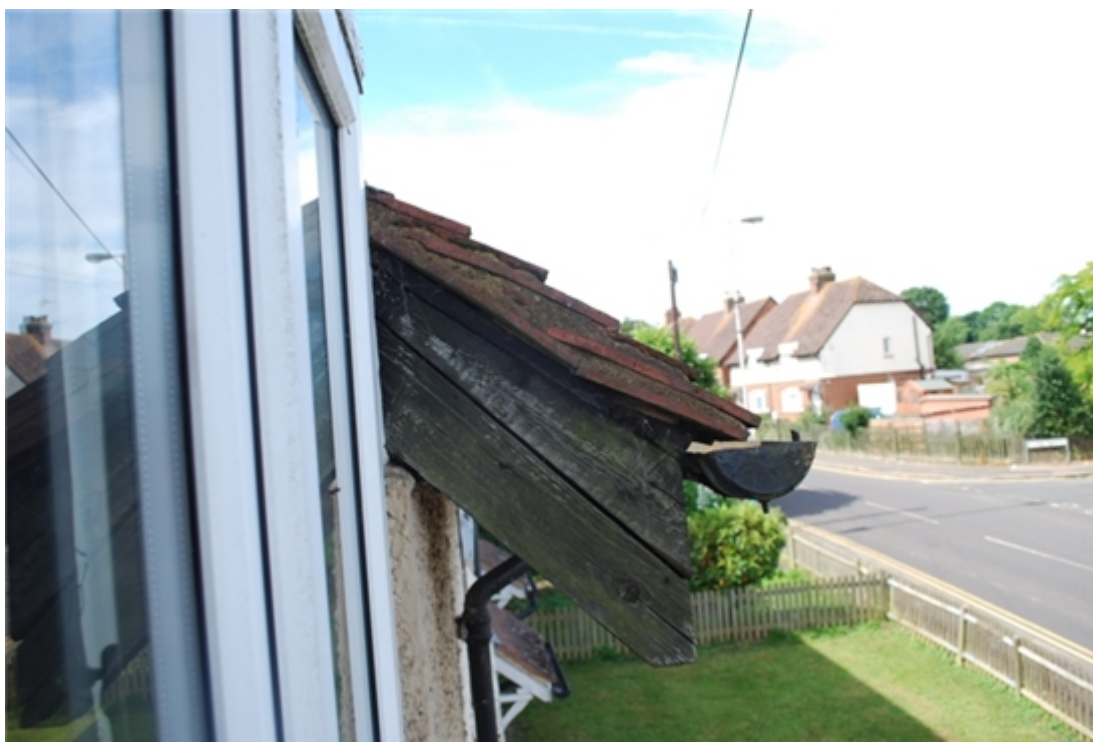
Roof joist decay.
