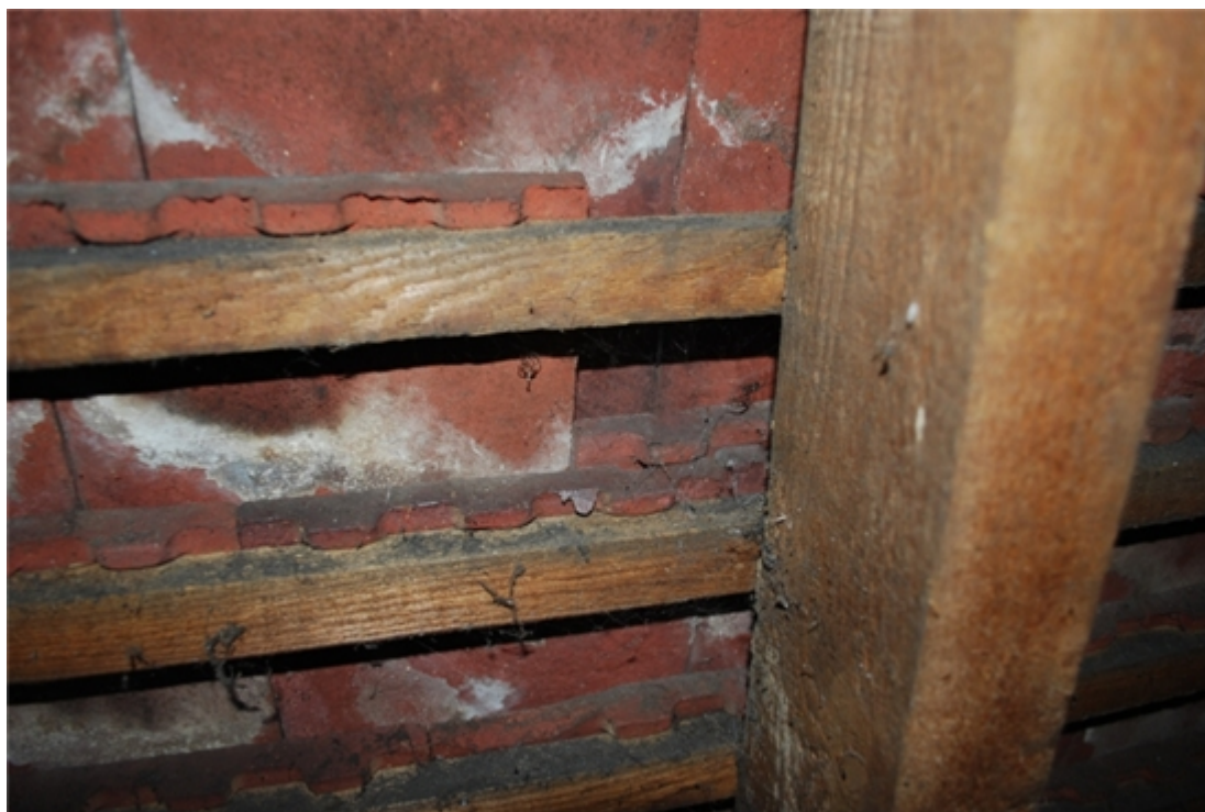
Slipped tiles visible in roof space.
